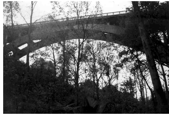
Figure 21 Grafton Road Bridge
