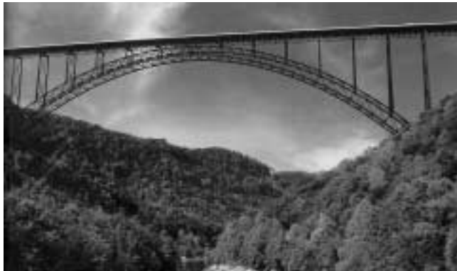
Figure 27 New River Gorge Bridge
