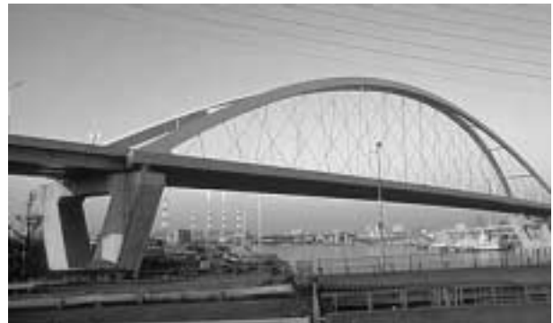
Figure 30 Shin Hamadera Bridge
