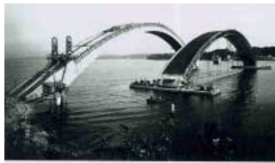
Figure 23 Floating Formwork for Plougastel Bridge
